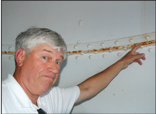
Roger Horton of the Lighthouse Committee points to corroded seams on interior walls.
